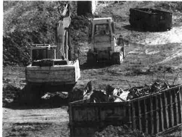
Construction waste should be collected in designated waste collection areas on-site, such as metal dumpsters.
